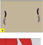
Mark the pipe clamp distances properly with 1% inclination on the wall or ceiling where they will be installed. (as flat wall)
